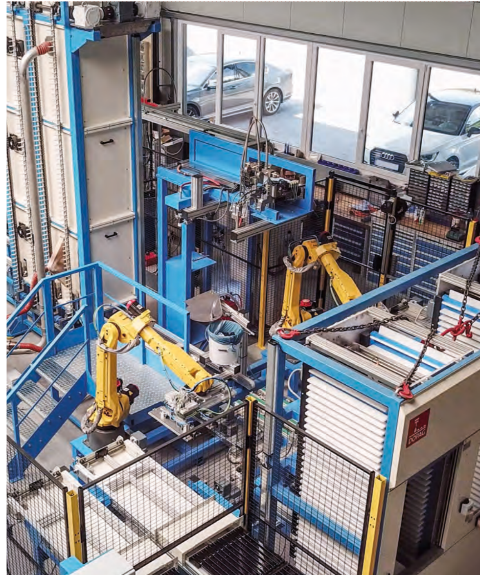
A custom-built dispensing system for the household appliance manufacturer Amica: Oven door components are being processed, including pretreatment with Pyrosil and post-treatment in a curing buffer.
